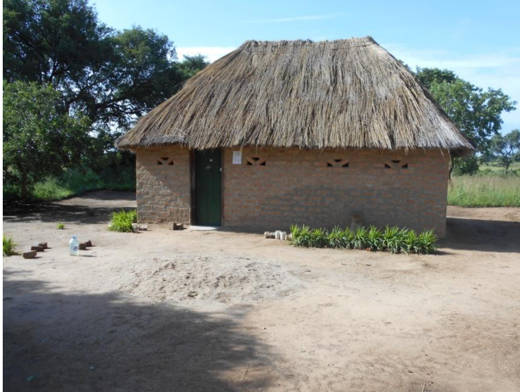
The SSAAP office/house completed.
