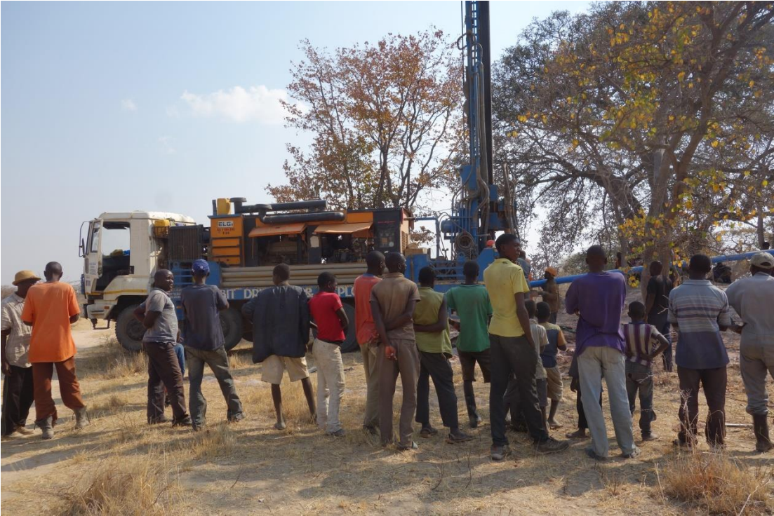
They pull the drilling pipes out of the ground and replace them with PCV casing pipes, then inside of the PCV pipes the pump stems which, when pressurized through the hand-pump, activates the water to come from the ground and exit the hole via the hand-pump at the ground level.
