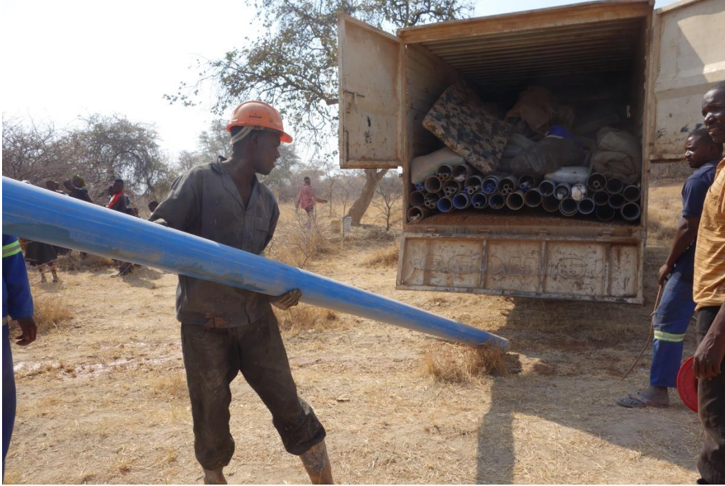
They pull the drilling pipes out of the ground and replace them with PCV casing pipes, then inside of the PCV pipes the pump stems which, when pressurized through the hand-pump, activates the water to come from the ground and exit the hole via the hand-pump at the ground level.
