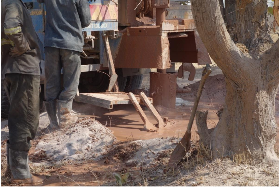
This site is going to have a very strong water source. We found water at 85 metres, but when they flushed the hole, found that it was filling up quickly (replenishing) and at only 22 metres, the water was available!
