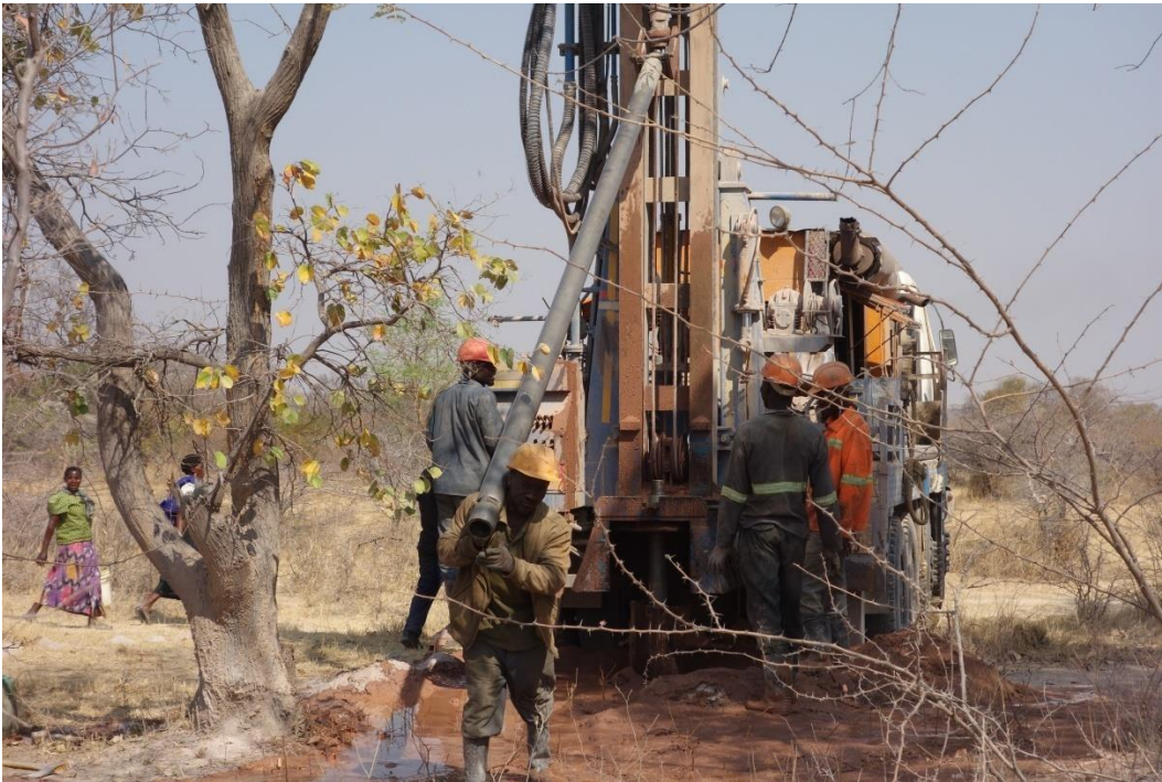
This site is going to have a very strong water source. We found water at 85 metres, but when they flushed the hole, found that it was filling up quickly (replenishing) and at only 22 metres, the water was available!
