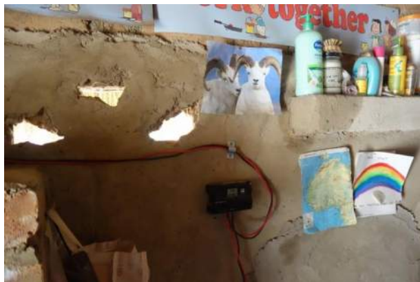
This device ensures that the power from the sun hitting the solar panel doesn't overcharge the battery thus ruining it.
