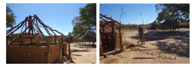
**Foundation of House**: This layer is made of a long piece of string ('*lozi*'), made of tree fibers, wrapped around sticks, stuck in the earth around all four corners of the perimeter of the house. The sticks and *lozi* compose the foundation for the house as its perimeter; the
