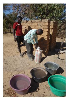
After the foundation is laid, the sides of the walls are laid with bricks and a mud-watergravel paste. This 'paste' is prone to termite damage, thus for homes that have the means as well as a long-term sustainability mission (such as the SSAAP Headquarters) it is preferable to mix cement with the mud paste – not only for the durability, but also to deter termites from entering. Doorway is built into one area of a wall. This process usually takes 1-2 days, needs 3-5 men to complete.
