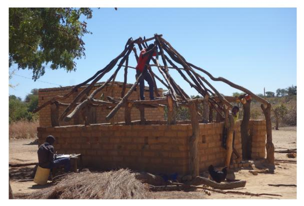
The houses in the village, unless made specifically with an iron sheet (*'malata'*) roof, are made entirely of earth; earthen materials include molded bricks, paste between bricks, wooden planks for the roof, roof made of dried grass, door and door frame are as well made of trees.
