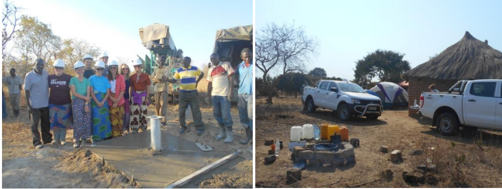
The EWB-MSU Team working with SSAAP in 2014. Left: The Team standing around the completed borehole in Siamabwe Village, Simwatachela Chiefdom, Southern Province, Zambia. Leonard, in yellow and blue stripes, was the contact person for this borehole. Right: More activity surrounded the SSAAP Center in a few short weeks than it will see for years!
