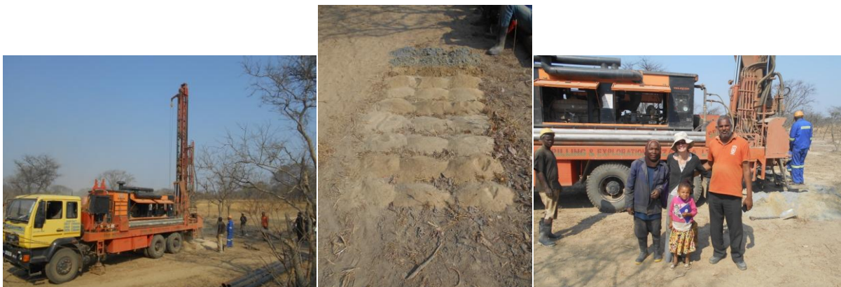
SRR Waterwell Drilling & Exploration Company's drill rig (left); notice the dryness in the land around the Simapuka site. Center: gradations of soil as it changes from sand to clay, then finally to mud – and darkens as it does so. Right: Mr. M. S. Reddy, Managing Director of SRR Waterwell Drilling & Exploration Co. at the Simapuka site on October 15, 2014.
