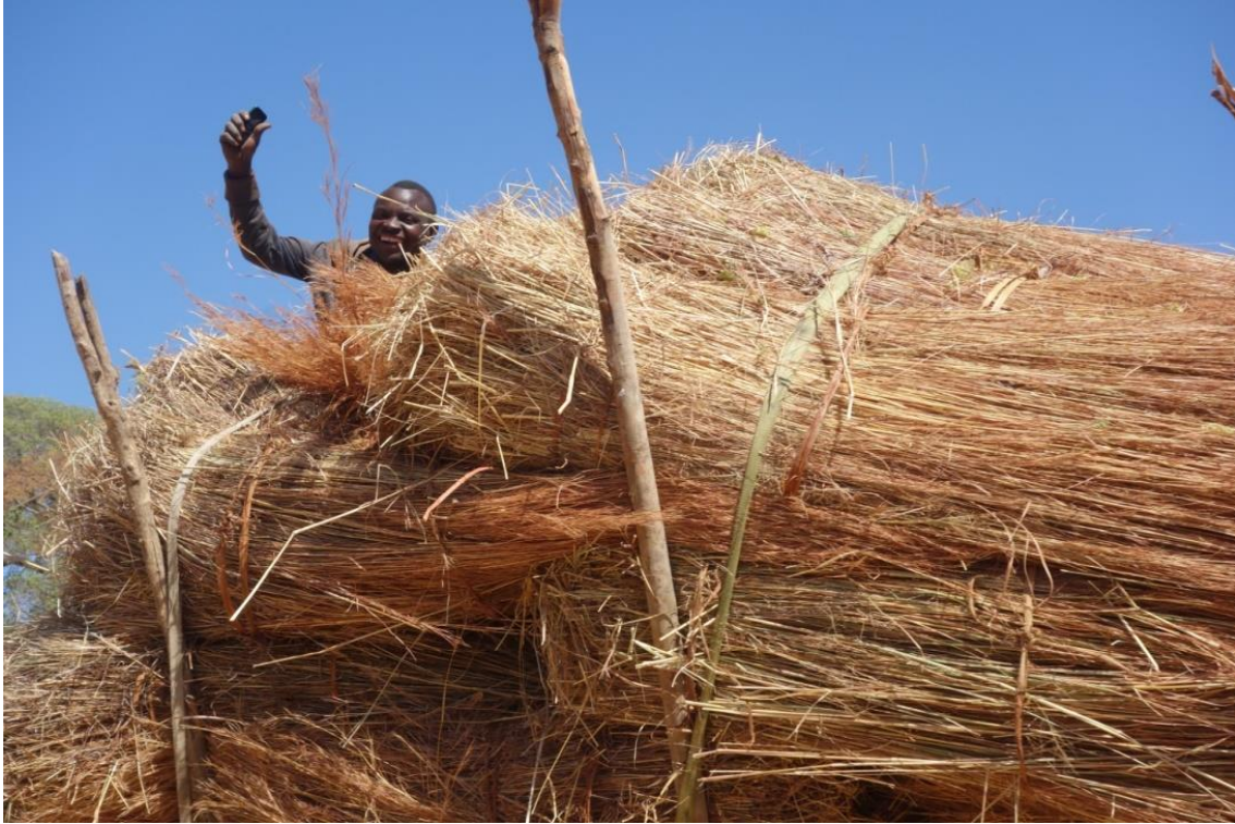
The arrival of our new roof! On the 10 th of September 2020.
